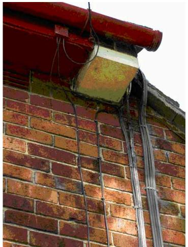
Later, a more detailed conversation with the homeowners revealed the cables to be the domestic supply cables for the property. They ran the full length of the front of the house at eaves level before dropping down to the wall to enter the meter / distribution box. A further set of cables continued to supply the farm outbuildings and milking parlour.
